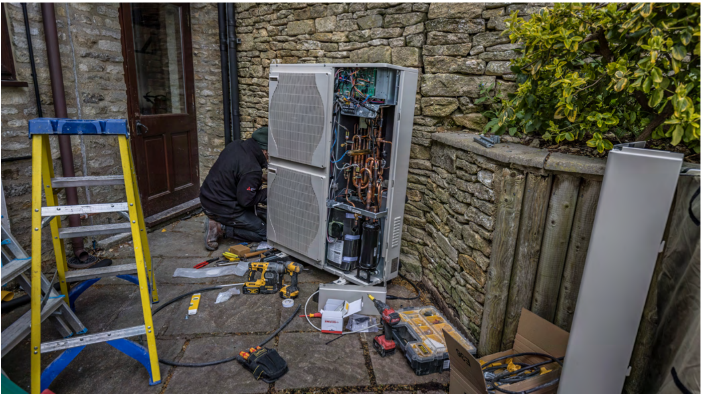
An air source heat pump being installed. Courtesy Cotswold Energy Group.
