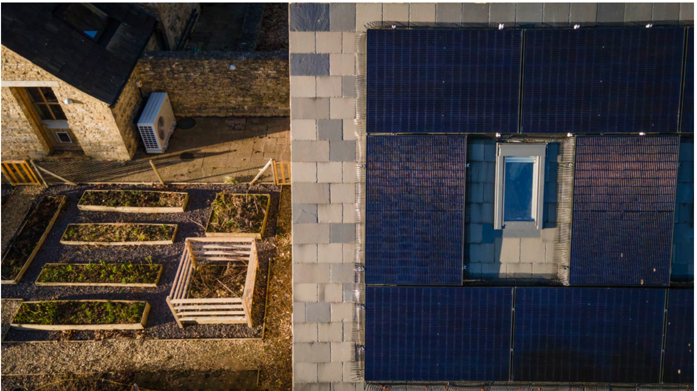
A building with a heat pump and solar PV. Image courtesy of Cotswold Energy.
