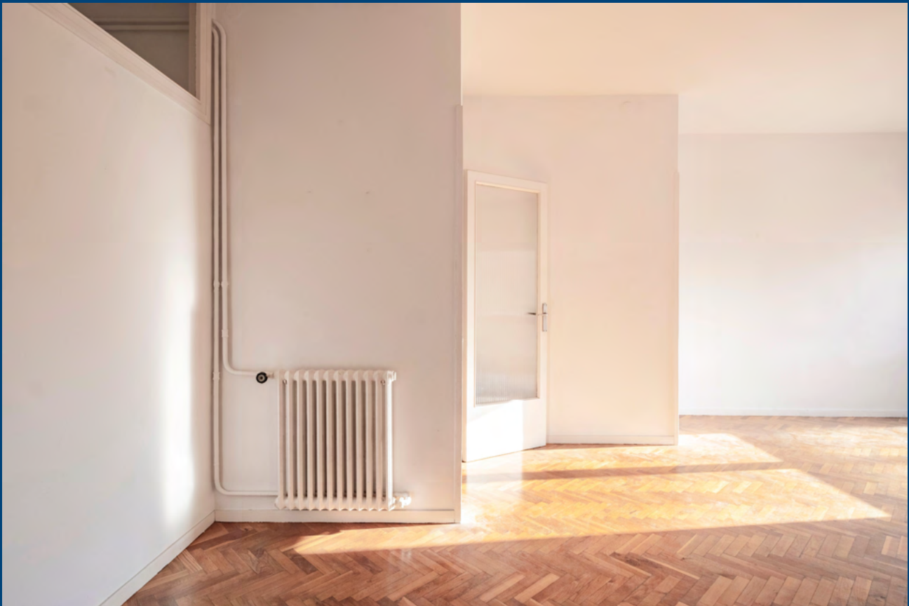
A radiator and associated pipework in a wet central heating system. Image from Shutterstock.
