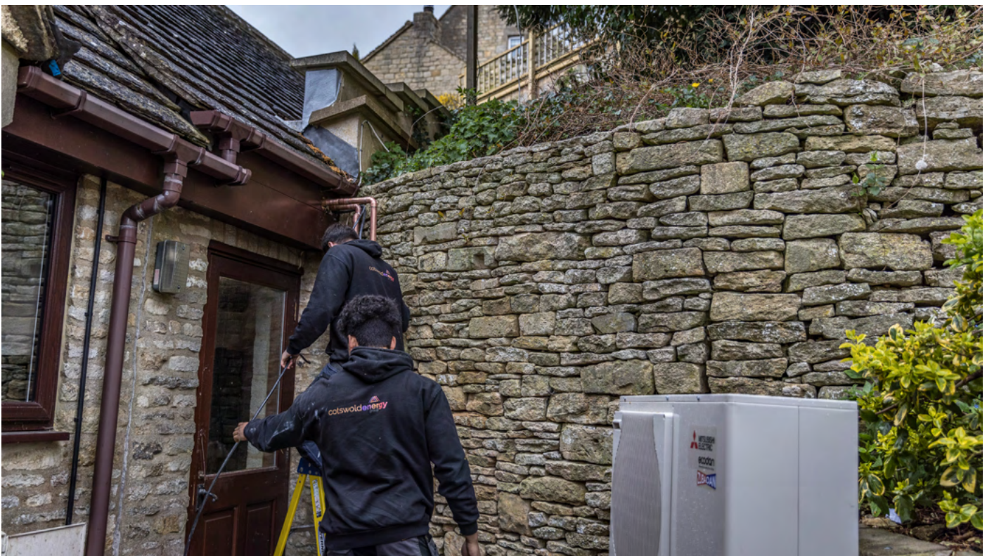
An air source heat pump being installed. Courtesy Cotswold Energy Group.
