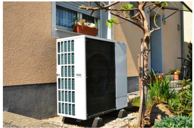
An air-source heat pump outside a home. Image courtesy of CLASP.
