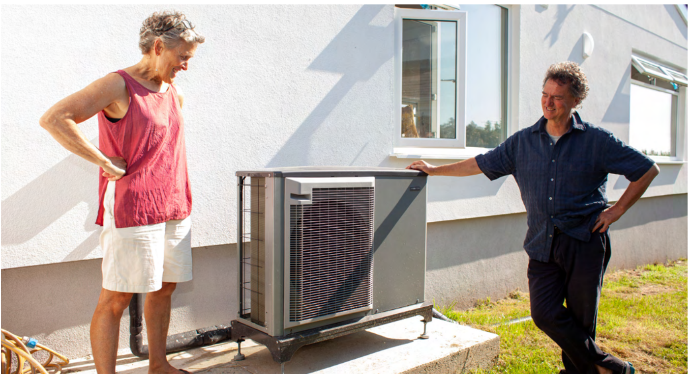
A domestic air-source heat pump. Image provided by Jonathan Atkinson, aka @lowwintersun.
