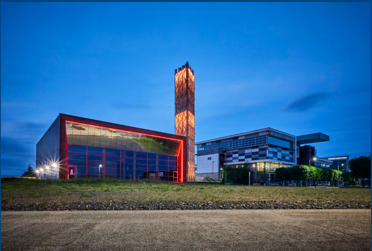
Queen's Quay 5.2MW water source heat pump, Glasgow, Scotland. Image courtesy of Star Renewables.
