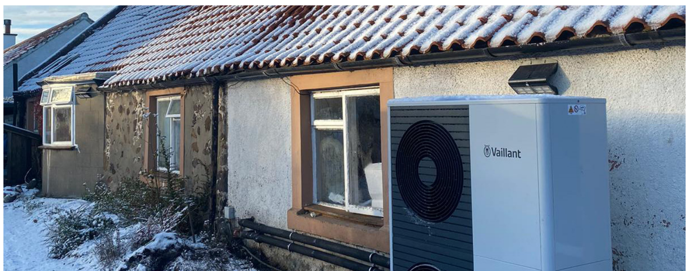
An air source heat pump during a cold spell. Courtesy of IMS Heat Pumps.
