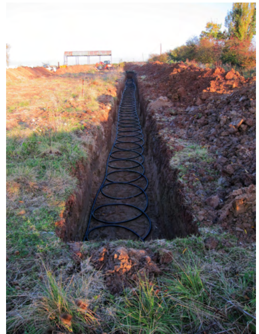
Left: Air-source heat pumps in situ (image courtesy of Joe Smyth). Right: A Slinky-style ground-source heat pump ground array (image courtesy of David Brooke). Images reprinted with permission.
